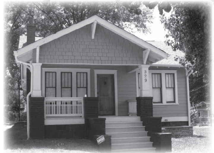
329 Park Avenue, Wilmore neighborhood.
