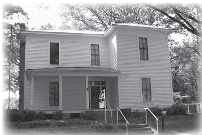
Dowd House, which served as the command center for the World War I training facility. Photograph courtesy of David Aaron Moore.
