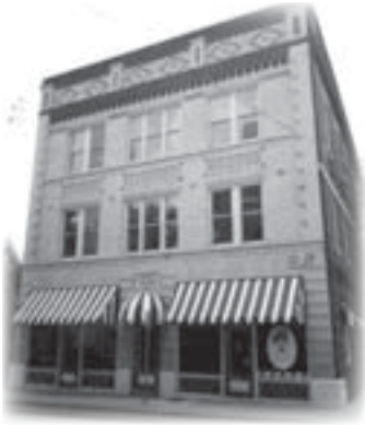
Mecklenburg Investment Co. Building (1922)
